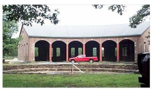
For this historical project in **Windham**, we provided the structural design of reinforced masonry walls and a wood & steel frame roof, all supported on the existing roundhouse foundation.
