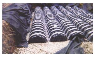
With the increasing concern for storm water runoff impacts of proposed developments, underground infiltration facilities are becoming more and more common. Here is an "Infiltrator" drywell bed being installed at one of our recent projects in **East Hartford**.
