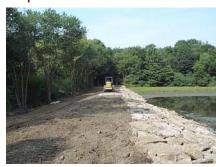
The repairs to the Lake Wackawanna Dam, in Danbury, are nearing completion. The concrete spillway has been finished, the stone masonry work is done, and the riprap slope protection is installed. A little fine grading, fence installation, and seeding and this dam will be "good to go" for a long time to come. This repair project is a joint effort of the Juniper Ridge Taxing District and the Connecticut Department of Environmental Protection.
